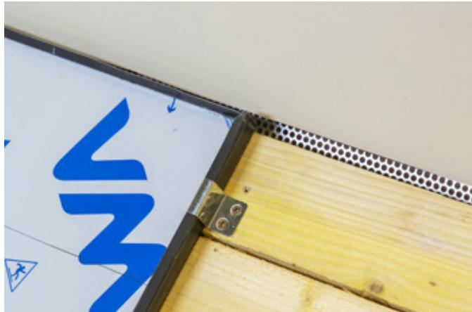
**NB :** For faster installation of the clips, do not crimp the seam too tightly at the wall ridge.
